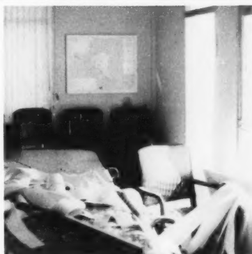
Damage inside the ambassador's conference room. (Photo by Tom Sullivan)
